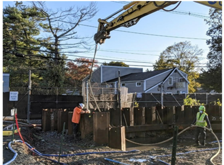
Installing Wellpoints for Dewatering
