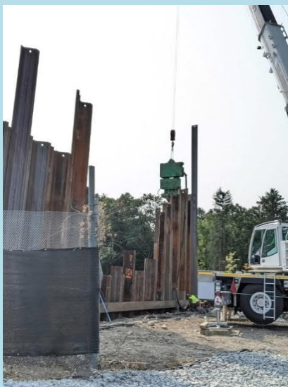
Installing Sheet Pile
