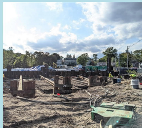
Sheet Pile and Bracing
